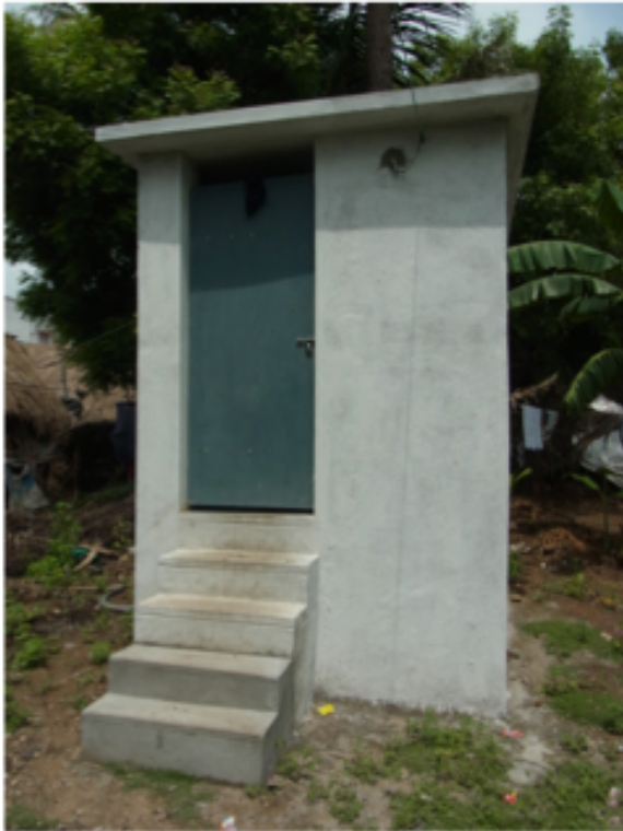
Double room EcoSan toilet in Bootheeri with light, shower and ventilation pipe
